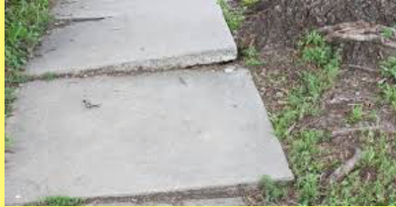
NEW OR REPLACED SIDEWALK
