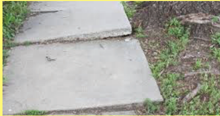
NEW OR REPLACED SIDEWALK
