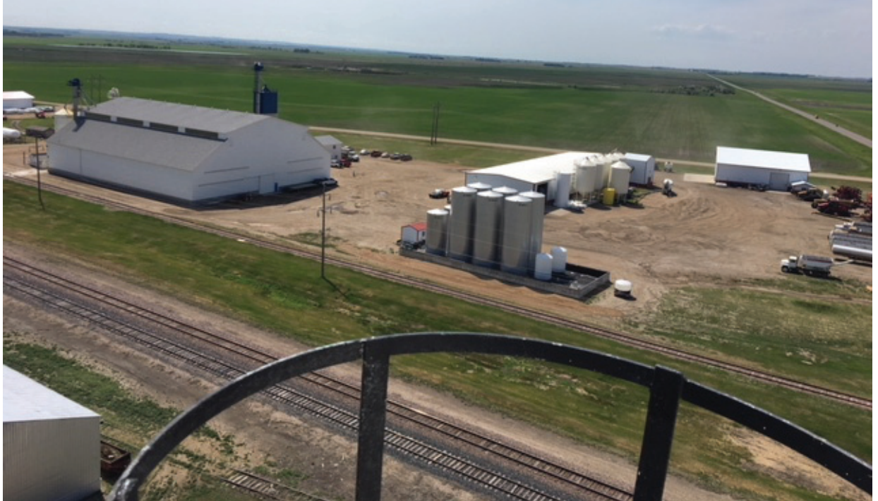
View to the south-east
