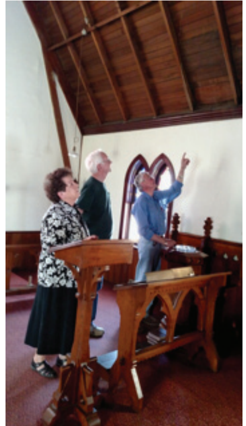
GCHS President "Topper" Tastad points to ceiling boards tacked over damaged roofing boards. (Courtesy Photo)
