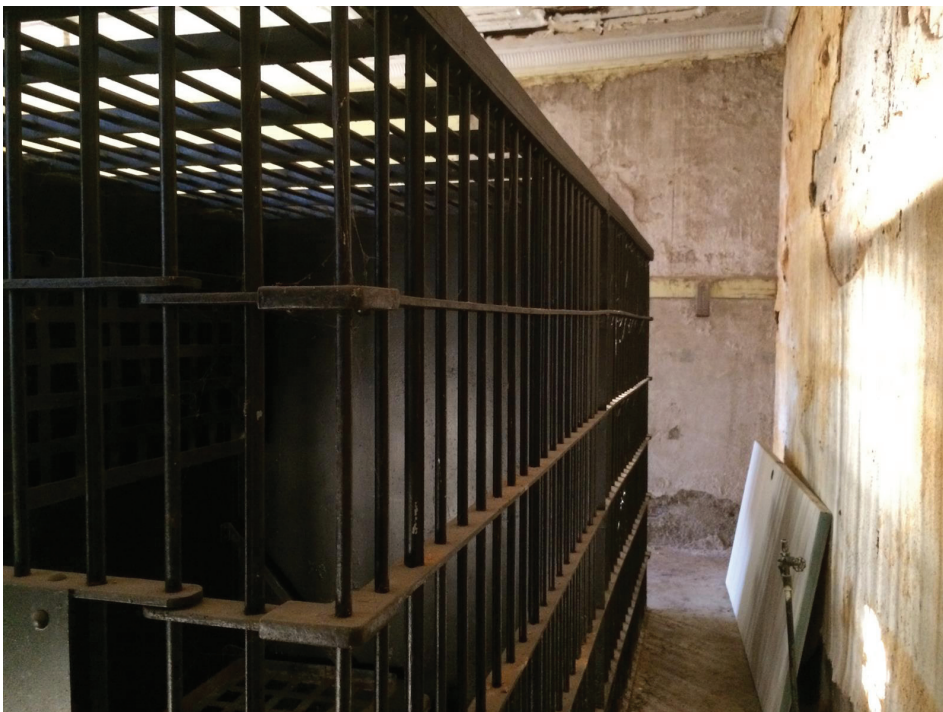
Left: This is the view of the inside of the jail building. (Photo
