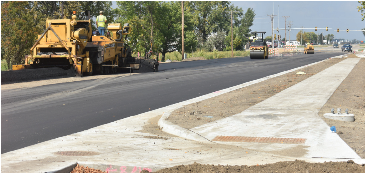
The long waited process of putting down asphalt on SD37 through Groton has begun. The first 1.5 inches of asphalt was laid down on Friday from US12 to Fifth Avenue. (Photos by Paul Kosel)
