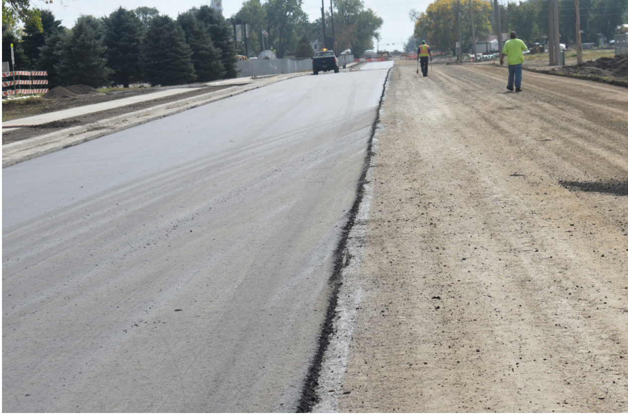
The long waited process of putting down asphalt on SD37 through Groton has begun. The first 1.5 inches of asphalt was laid down on Friday from US12 to Fifth Avenue. (Photos by Paul Kosel)
