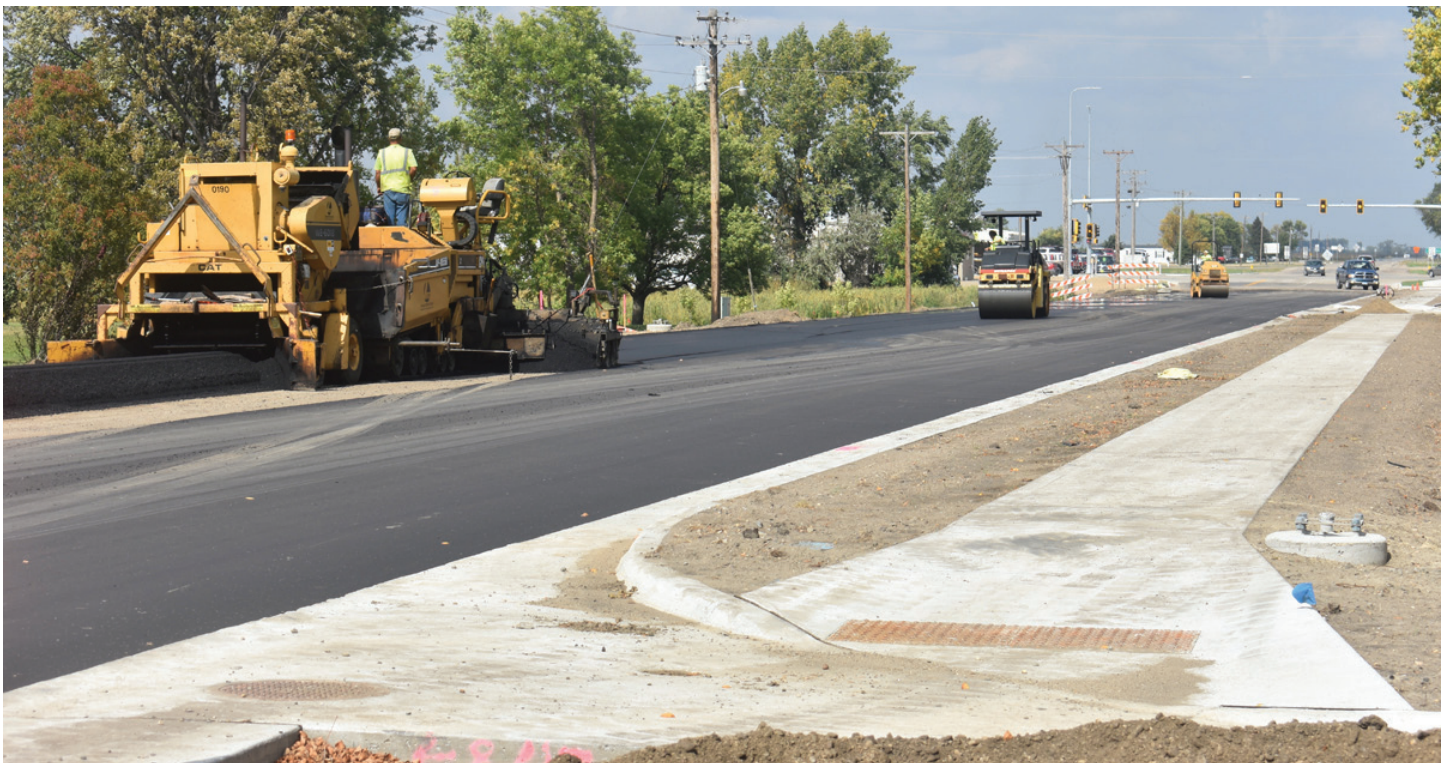
The long waited process of putting down asphalt on SD37 through Groton has begun. The first 1.5 inches of asphalt was laid down on Friday from US12 to Fifth Avenue. (Photos by Paul Kosel)
