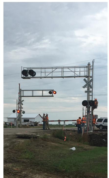
The new west signal light and arm was installed on Tuesday. The east one is scheduled to be installed on Wednesday.
