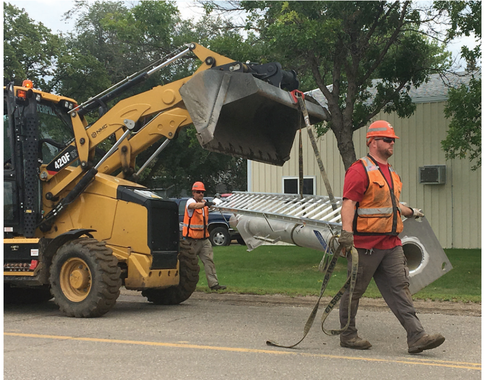
Burlington-Northern Railroad workers were guiding a new crossing to its resting place. The railroad cross on the south edge of Groton is being replaced as part of the highway project.
