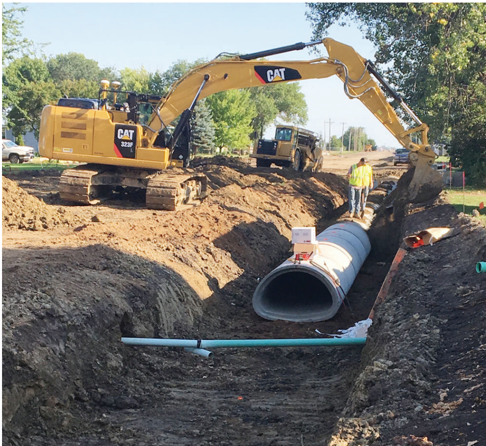
As you can see in this photo, the sewer service line is a little too high for the big storm sewer pipe that is being installed. At least four homeowner sewer service lines had to be removed and reinstalled about 18 inches lower to accommodate the new concrete storm sewer.
