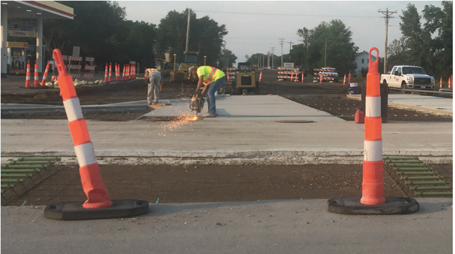
Saw cuts were being made on the concrete road Saturday morning.
