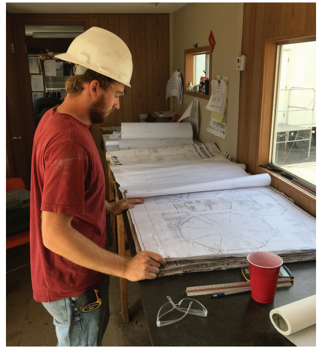
Tyler Hollinsworth was the acting superintendent for JDH Construction on the day GDILIVE.COM was filmed last week. He is reviewing the set of plans at the headquarters on the Groton Area Elementary School grounds. (Photo by Paul Kosel)
