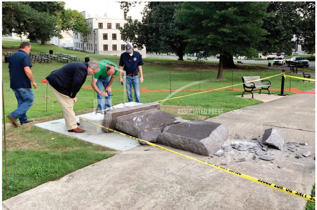
Personnel from the Secretary of State's office inspect the damage to the new Ten Commandments monument outside the state Capitol in Little Rock, Ark., Wednesday morning, June 28, 2017, after someone crashed into it with a vehicle, less than 24 hours after the privately funded monument was installed on the Capitol grounds. Authorities arrested a male suspect. (AP Photo/Jill Zeman Bleed)
