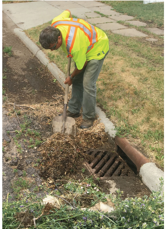
The city workers went through town cleaning out the storm sewer inlets. Many of them were completely plugged up with grass and leaves. Above is Aaron Severson and in the right photo is Brian Gravatt.
