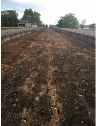
One pass the length of SD37 was milled up Tuesday. SD37 will be undergoing a transformation with new storm sewer, new curb and gutter, new street lights, a new road and new sidewalk from Railroad Avenue to US12 on the east side and from Railroad Avenue to Sixth Avenue West on the west side. SD37 will be out of commission for most of the summer.
