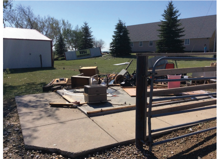
Threshermen's Park building (Andover) removed from foundation and moved over 100 feet.
