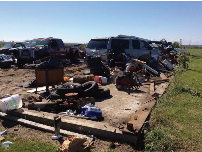
Metal outbuilding removed from foundation 1 mile east of Andover
