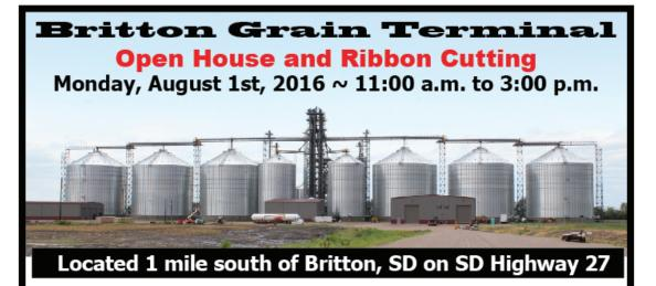
This recently completed facility has a licensed capacity of 4.5 million bushels of upright storage. In total, the new facility will be capable of receiving grain at 60,000 bushels per hour and loading 120-car shuttle trains at 80,000 bushels per hour.
