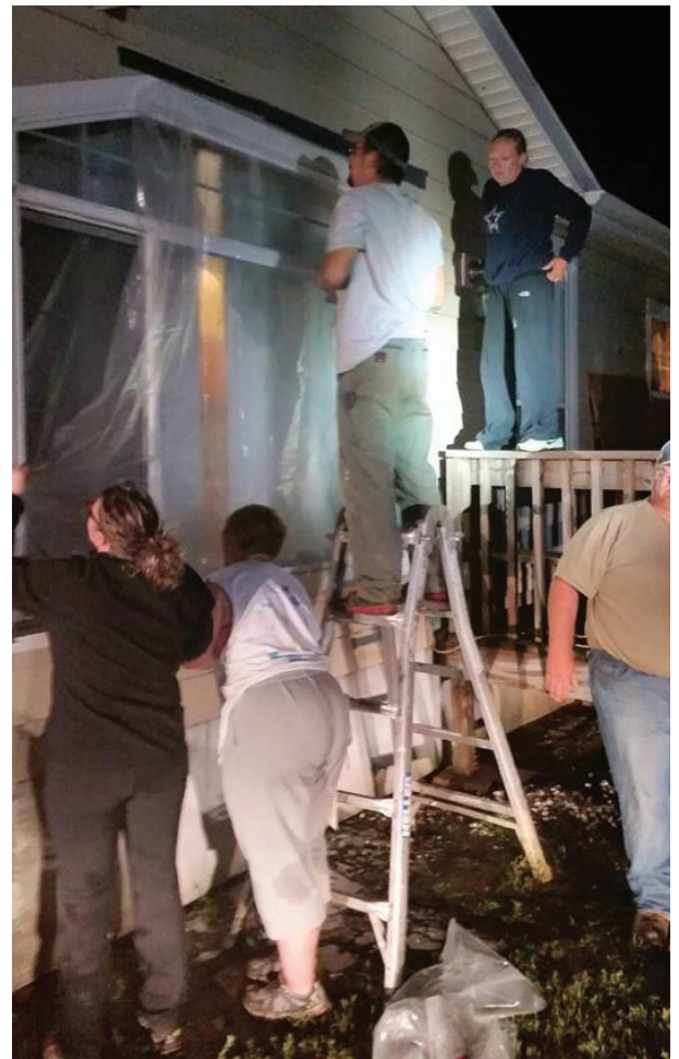
Neighbors came over to help put plastic over the windows. (Facebook Photo by Michelle Johnson)
