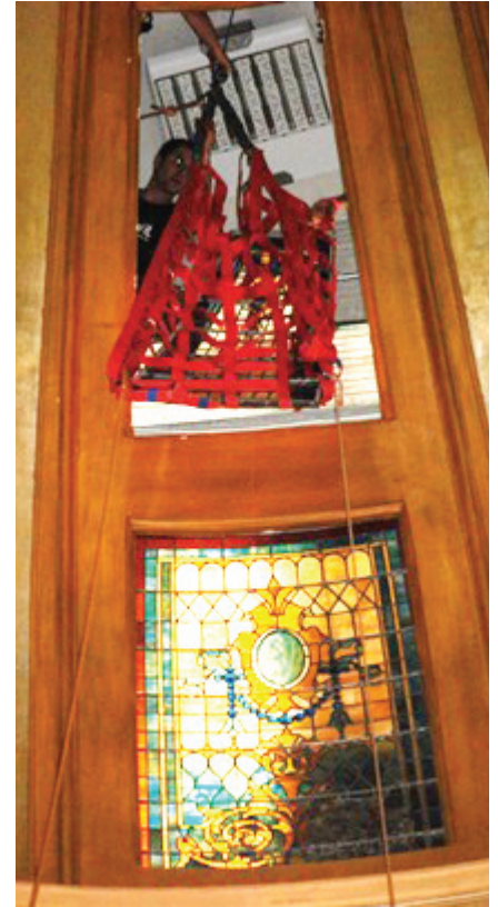
* A panel of restored stained glass being reinstalled in the Capitol.
