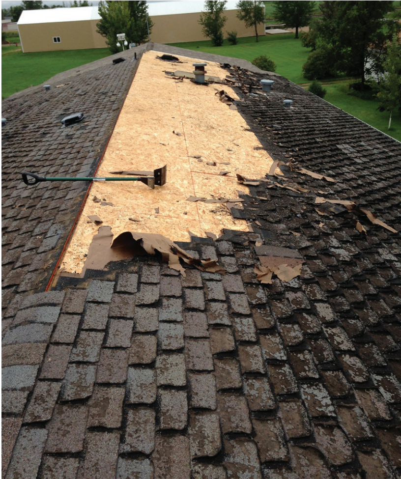
Above Photo: The deshingling of the west side of the roof began. The photo below shows the almost completed roofing project. The top right photo features Paul Kosel tearing off the old shingles.
