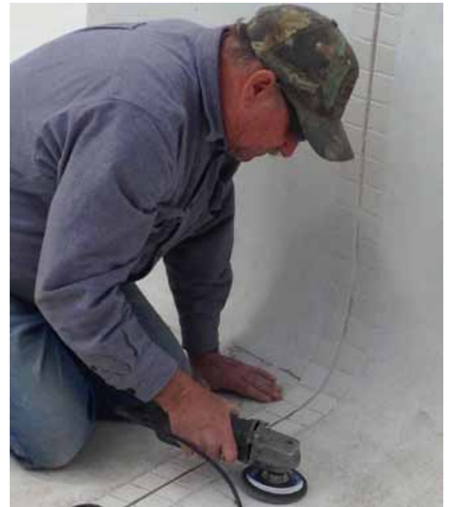
Jim Thom from Associated Pool Builders, Bismarck, was here on Wednesday to file down the rough spots at the Groton Swimming Pool. Two tiles also had to be replaced and the filling of the pool will begin tomorrow.
