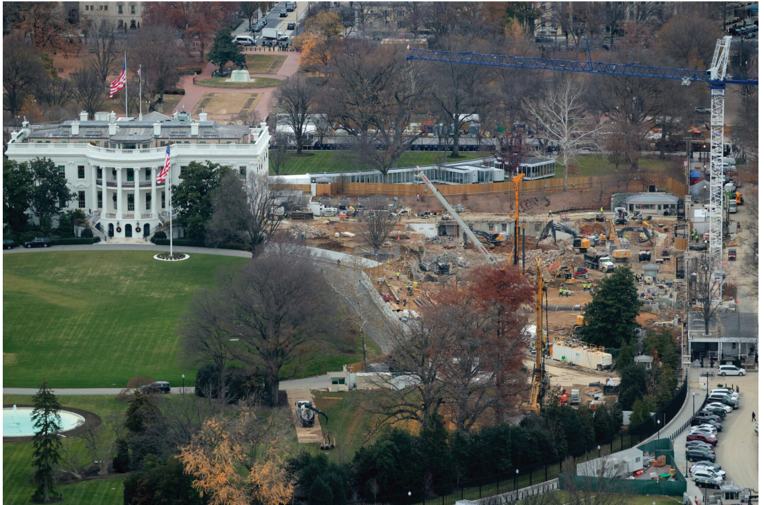
Demolition work continued where the East Wing once stood at the White House on Dec. 8, 2025. President Donald Trump ordered the 123-year-old East Wing and Jacqueline Kennedy Garden leveled to make way for a new 90,000-square-foot ballroom. (Photo by Chip Somodevilla/
