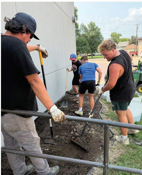
Aaron Severson, Nick Groebelinghoff (in back), Alex Abeln and Gavin Englund are removing rock from the north side of the building.
