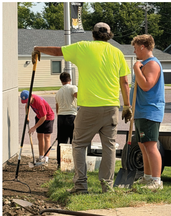
Nick Groebelinghoff, Donavan Block, Aaron Severson and Gavin Englund are busily removing the rock from the east side of the building.
