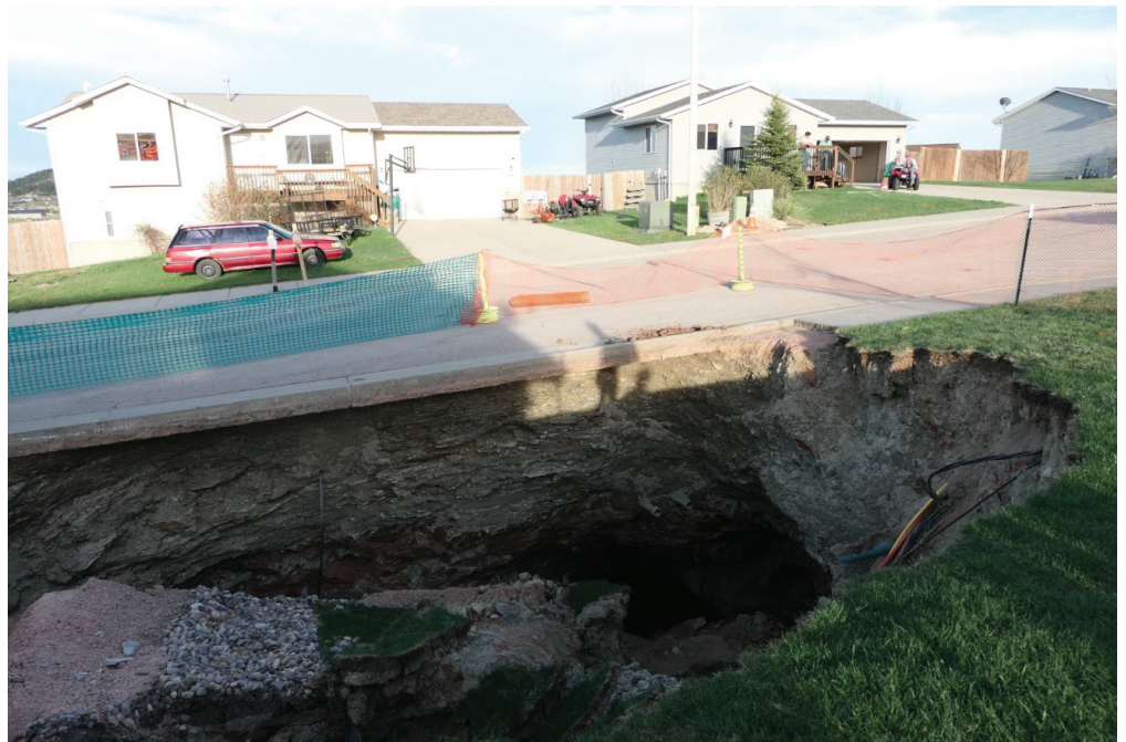
A spring 2020 view of a sinkhole in Black Hawk that opened near homes built atop a former gypsum mine. (Courtesy of Dan Austin)
