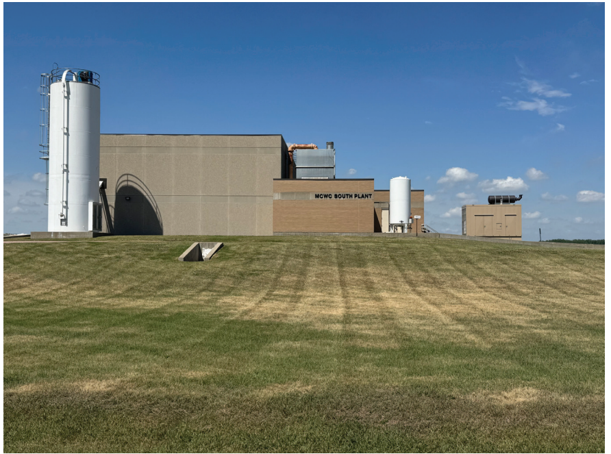
The existing water treatment plant for the Minnehaha Community Water Corp. is located south of Dell Rapids, S.D. (Photo: Bart Pfankuch / South Dakota News Watch)
