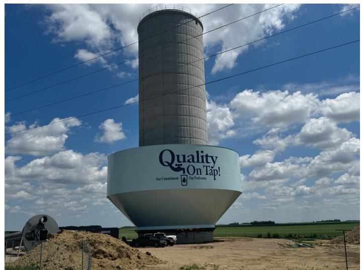
A 1.5 million gallon water tower was under construction in early June 2026 as part of the Shared Resources expansion effort by two rural water systems. (Photo: Bart Pfankuch / South Dakota
