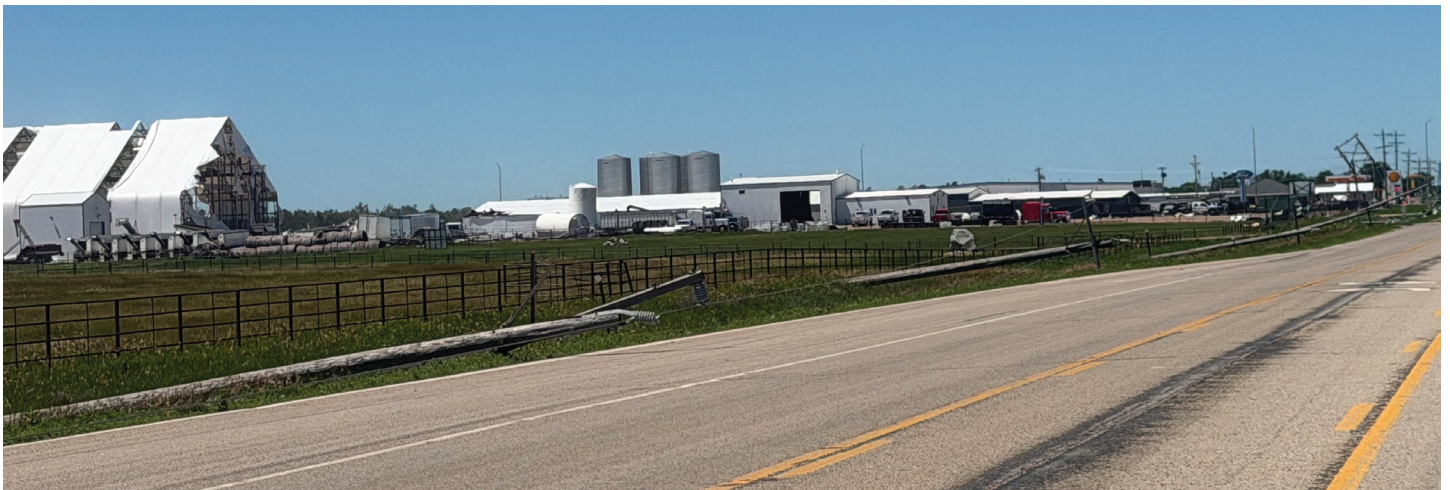
The town of Highmore was devastated with damage as 131mph wind whipped through the city on Monday. (Photo by Paul Kosel)
