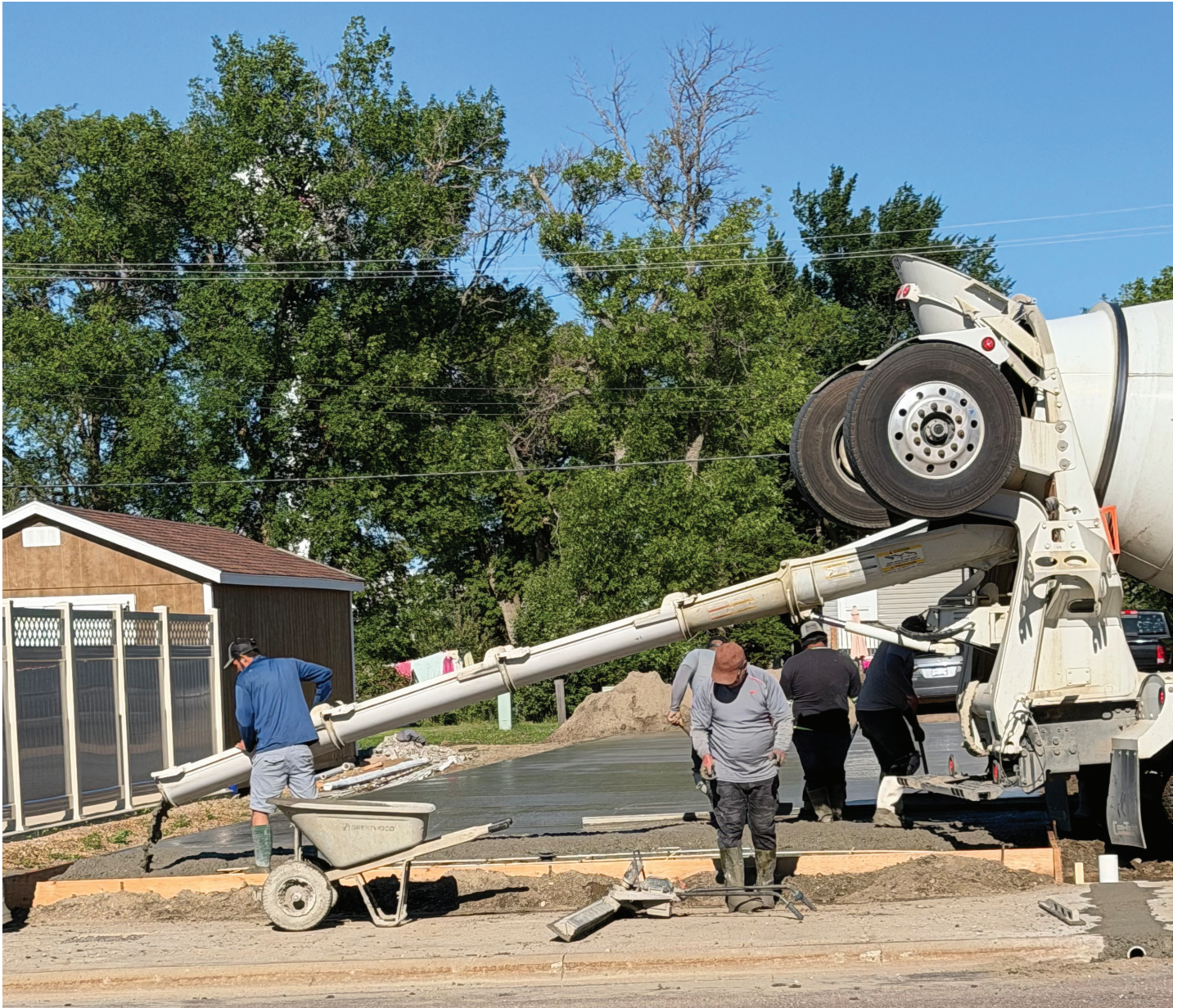
The concrete was poured on Tuesday for the new 10-stall garage going up just north of the Groton American Legion. (Photo by Paul Kosel)
