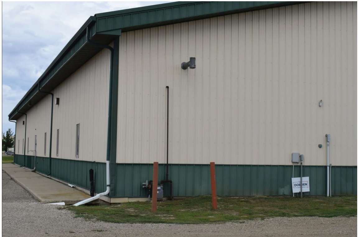
A building at 605 East Drive in Aberdeen, S.D. on June 15, 2026, which was zoned for 150 bitcoin mining units in 2022 by Plaza Rentals and Doeden's son Jonathan. (Photo: Molly Wetsch/South Dakota News Watch)
