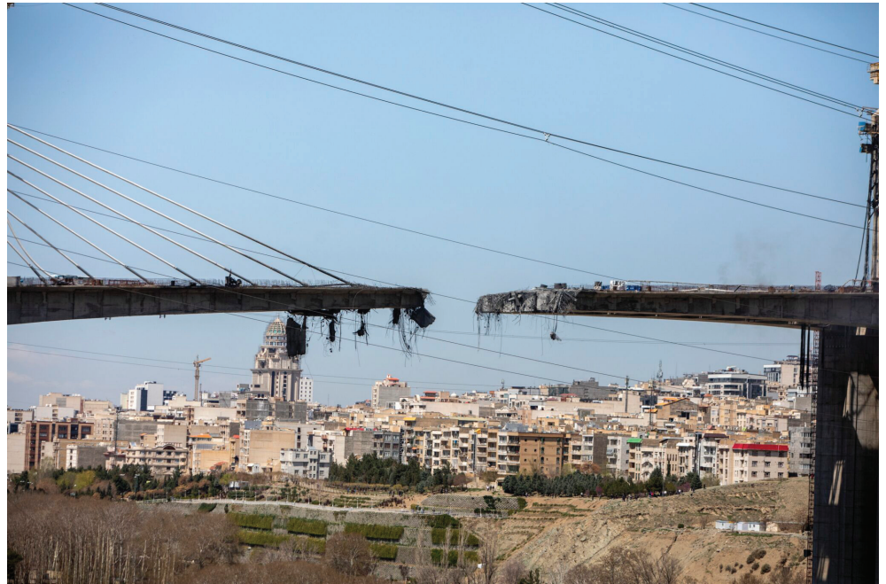
A view of the damaged B1 bridge, a day after it was destroyed by an airstrike, on April 3, 2026 west of Tehran in Karaj, Iran.
