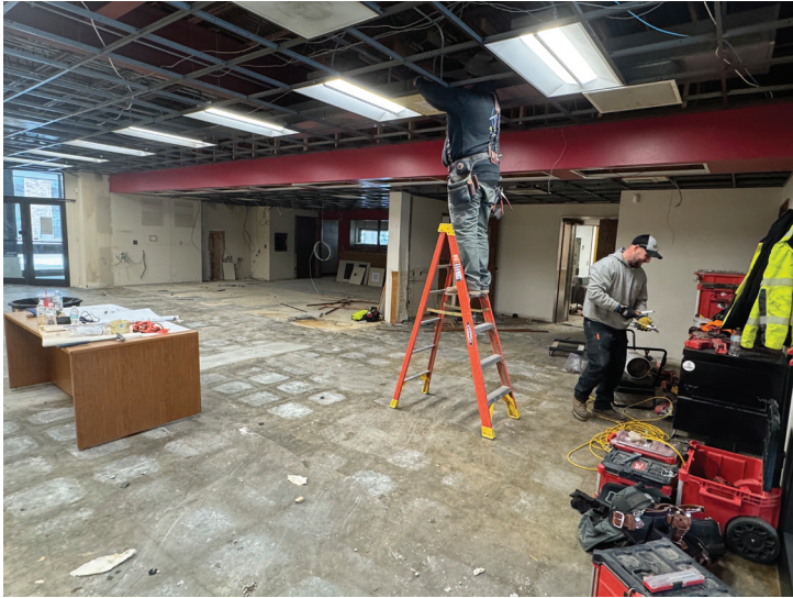
Work on the interior of the new daycare.
