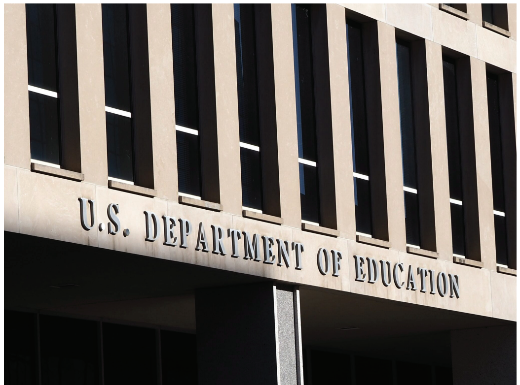
The Lyndon Baines Johnson Department of Education Building on Nov. 25, 2024. (Photo by Shauneen Miranda/States Newsroom)
