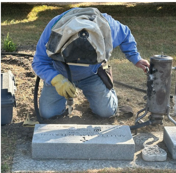
Rausch applies 100 psi to the stone to carve out the date.
