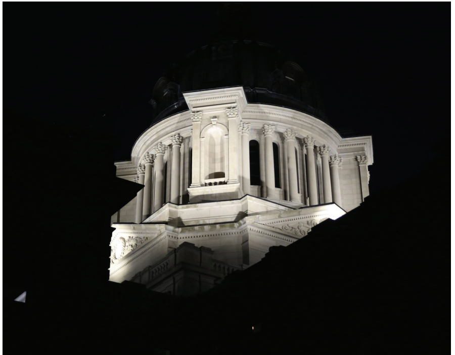
The South Dakota State Capitol at Pierre in December 2024. (Makenzie Huber/South Dakota Searchlight)
