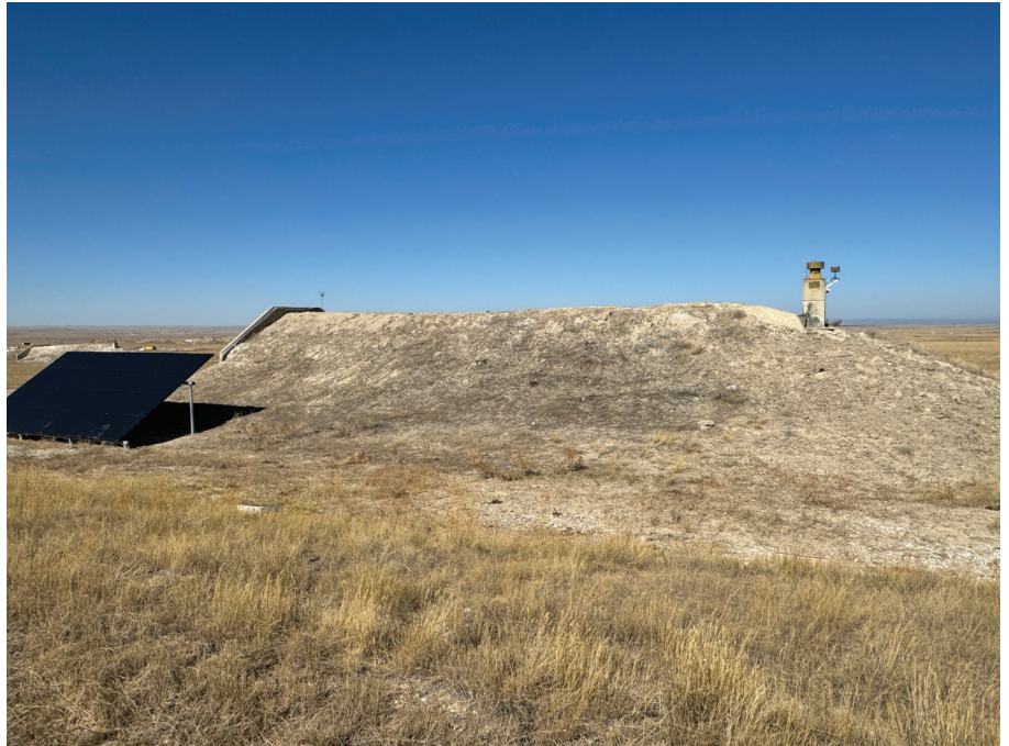
A bunker in the Vivos xPoint complex, shown on Oct. 4, 2024 near Igloo, S.D., has a solar panel and ventilation pipe in place. (Photo: Bart Pfankuch / South Dakota News Watch)
