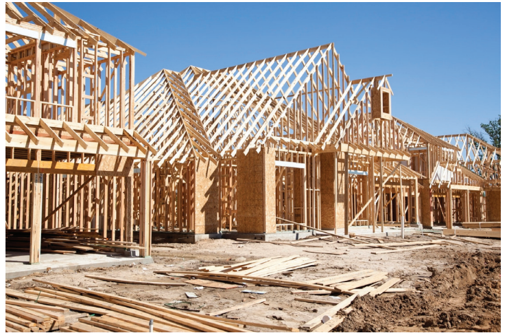
Houses under construction. (Getty Images)
